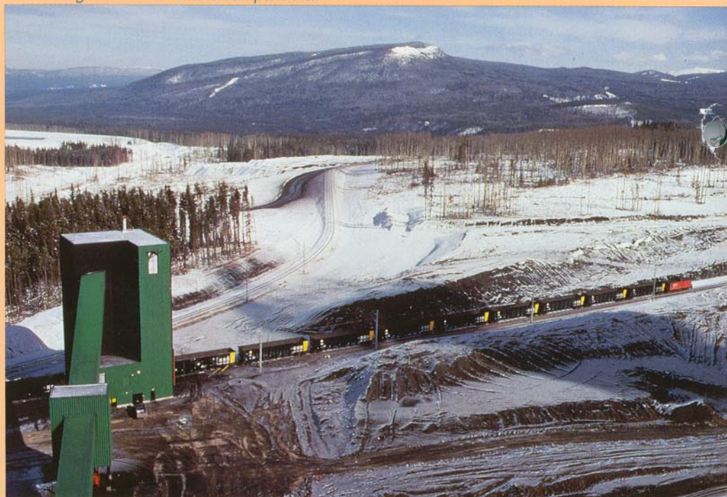
A PEBCO® coupled-in-motion system serves this large coal mine with 8000 TPH capacity.
